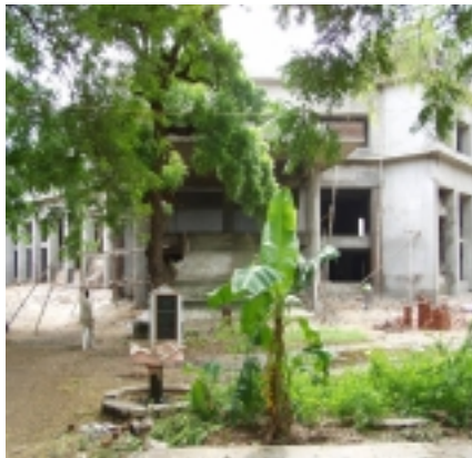
Front entrance to the Auditorium (Picture received Sep 28, 2003). Visit www.photos.gmcana.org for more recent ones.
